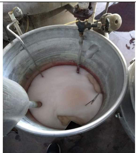
Photo: Colour and Chemical addition tank
